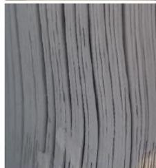
This photo shows a filter cartridge that should be cleaned. Keeping the pleats visible is key to moving air from the cabinet. Moving air means cabinet visibility and pleats still showing means air is being moved.
